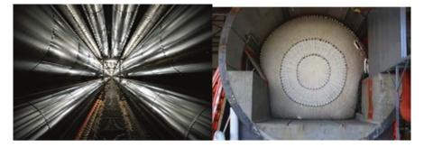
**Fig. F.90** (left) Utility tunnel for district heating pipes between Rigshospitalet and Amagerværket in Copenhagen, (right) tunnel plug developed by DHS S&T
