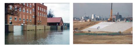
Fig. F.89 Masonry floodwall in Fargo, MD (left); armored levee in Japan (right)
