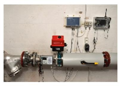
Fig. F.74 Dantaet pressure section (leakage protection)
