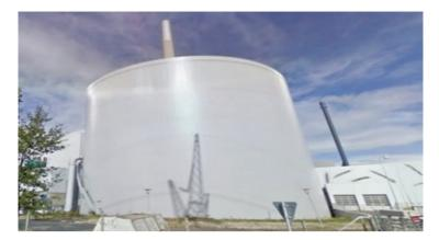
**Fig. F.52** The largest tank is probably the  $75,000 \text{ m}^3$  (2,648,600 ft<sup>3</sup>) pressureless hot water storage tank in Odense Denmark owned by Fjernvarme Fyn
