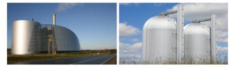
Fig. F.79 Viborg gas CHP with thermal storage and the thermal storage at Avedøreværket, Denmark
