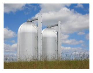
Fig. F.54 Thermal storage at Avedøre CHP plant
