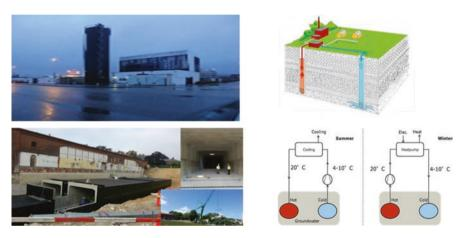
Fig. F.82 Steel tank, concrete chamber, and ATES
