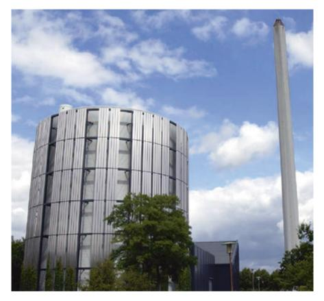
Fig. 7.17 Hot-water storage tank with a capacity of 8000 m<sup>3</sup> (2823 ft<sup>3</sup>), ready to use
