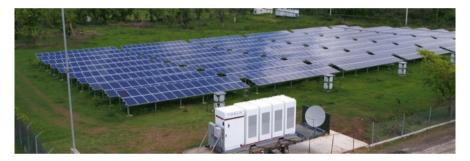
Fig. 7.10 Emergency power generation using a PV panel field connected to a battery pack
