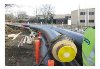
Fig. F.61 Installation of pre-insulated pipes
