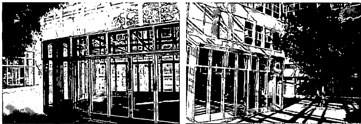
Figure 4.6.4 Atrium "East". Left: Inside view from back to front, through cafeteria building, still empty. Right: Inside view from front to back with cafeteria building and tree.
