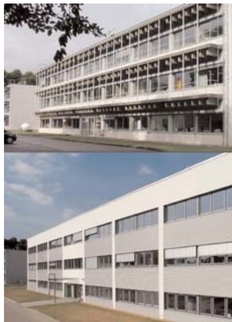
Figure 4-60: The laboratory building before and after refurbishment
