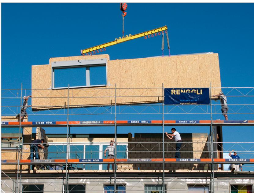
*Mounting a prefabricated, highly insulating façade element.*
