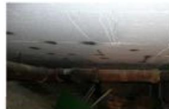
Figure 22: To ensure the best possible improvements and overall performance of the school's envelope thermal insulation was installed even on the commonly inaccessible ceiling below ground floor. [1]
