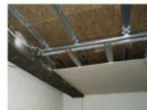
Figure 18: Installation of the insulation on the ceiling of the ground, space that is unconditioned.
