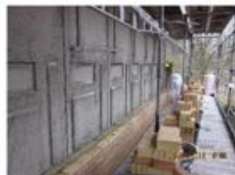
Figure 9 : New 190 mm insulation plus exterior solid standard bricks in the construction phase - shown with scaffolding
