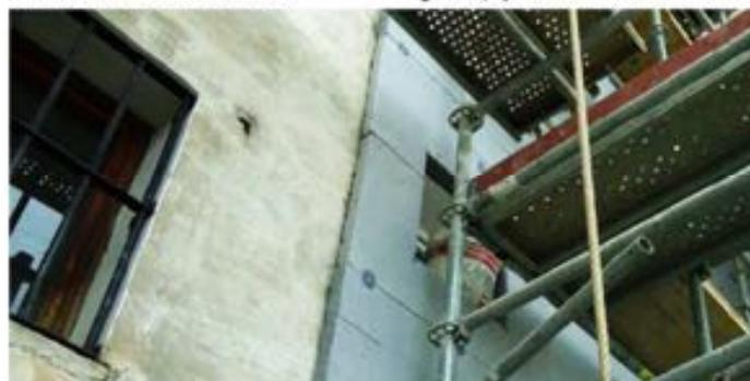
Figure 16: Installation of facade insulation, 6cm extruded polystyrene.
