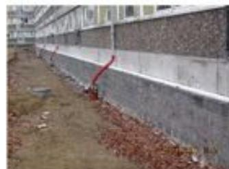
Figure 12: The external insulation of the basement covered by Leca bricks
