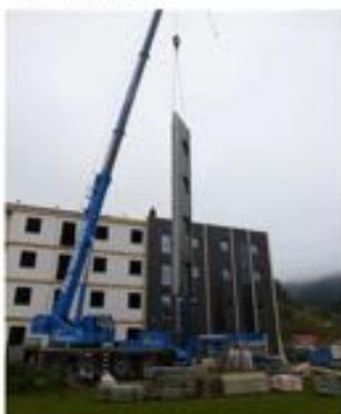
Figure 6: assembling of the prefabricated façade modules
