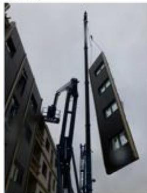
Figure 4: prefabricated façade element
