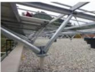
Figure 11: renovated flat roof with scaffold for the mounting of the photovoltaic panels
