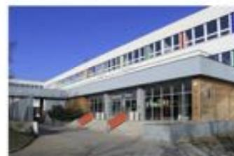
Figure 17: Main entrance of the school after renovation. Addition of (not heated) anteroom reduced heat losses through the entrance doors.
