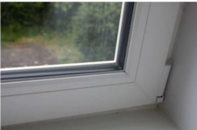
Figure 14: Lower corner of a plastic triple-glazed low energy window
