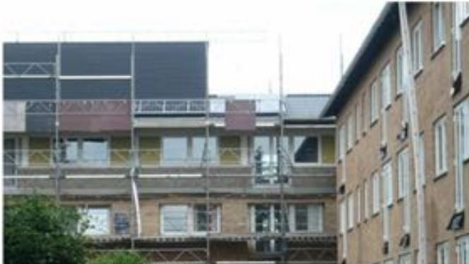
Figure 3: Retrofitting of exterior walls
