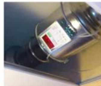
Figure 17: LeanVent damper in place on an air inlet duct to reduce energy consumption
