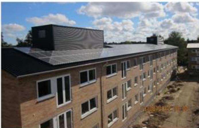
Figure 20: The 33 kW<sub>p</sub> south-facing PV system and the coverings for the new mechanical ventilation systems located above each stairway
