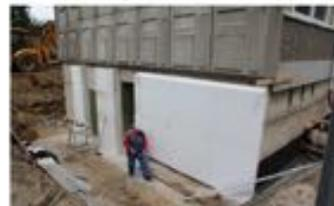
Figure 11: The external insulation (EPS) of the basement walls
