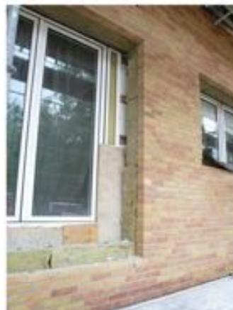
Figure 8: The new insulation and new windows almost in place
