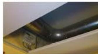
Figure 16: A new ceiling in the corridor is used to hide the inlet ventilation ducts
