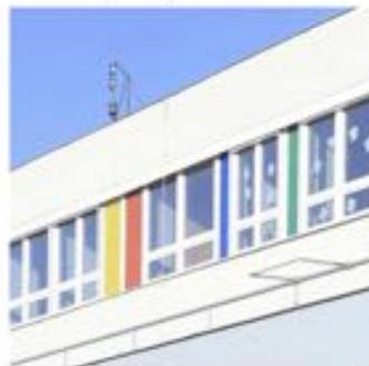
Figure 14: Row of windows (2nd floor) after renovation separated by colored plastic panels.
