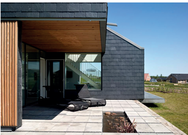
Shading (to reduce solar gains) and ventilation should be applied to reduce cooling loads and avoid overheating.
