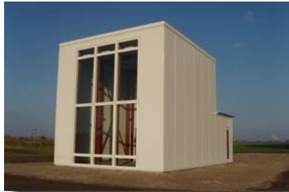
Aalborg University Double-Skin Facade Test Facility in Aalborg, Denmark
