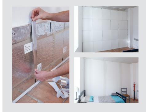
The installation process of the SLIMISOL system, consisting of a vacuum insulation panel with a protective layer and plaster board. Source: www.slimisol.fr
