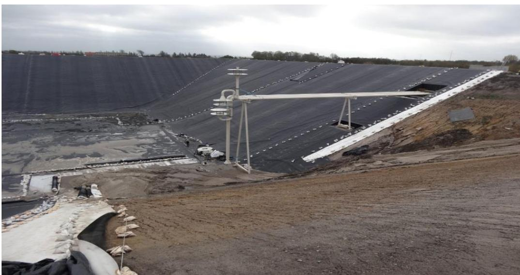
Fig. 4: Heat storage pit under construction
