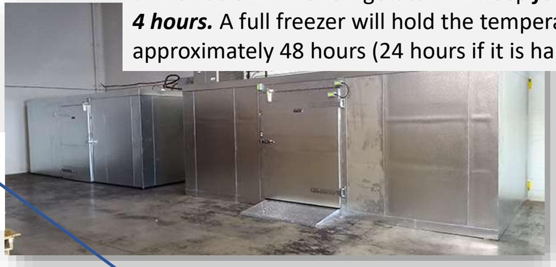
**Walk in Cooler.** To prevent food spoilage, the refrigerator temperature shall be at 40 °F or below and the freezer is at 0 °F or below. The refrigerator will keep *food safe for up to 4 hours*. A full freezer will hold the temperature for approximately 48 hours (24 hours if it is half full).
