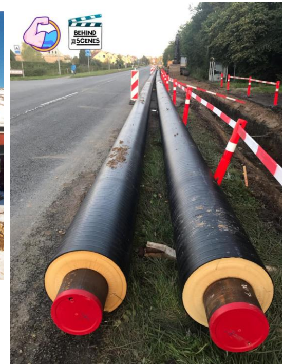
Direct buried pipe installation.
