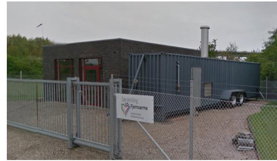
Portable district heating boiler.
