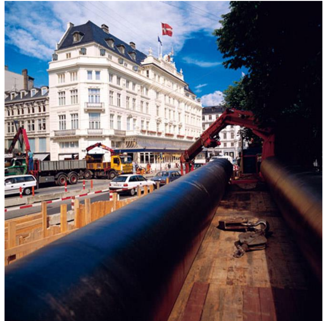
Installation of a pipe in central Copenhagen. Source: Danish Board of District Heating
