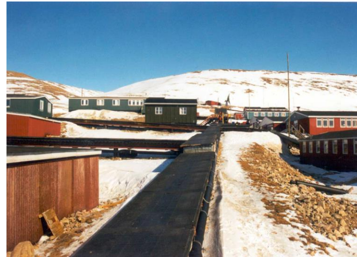
Pipeline in Thule, Greenland. Source: Ramboll A/S
