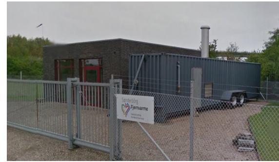
Portable district heating boiler.
