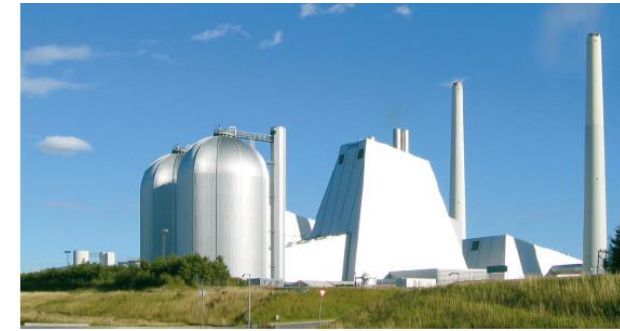
Thermal storage tanks. Source: Ramboll A/S
