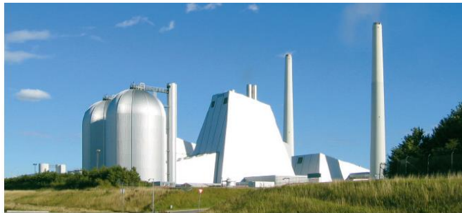
Thermal storage at a CHP plant. Source: Ramboll A/S
