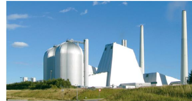
Thermal storage tanks. Source: Ramboll A/S
