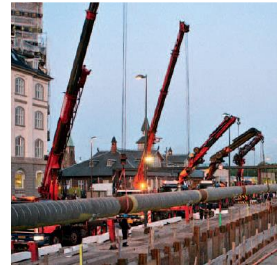
Installation of a pipeline. Source: Ramboll A/S
