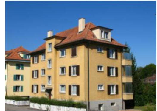
Simple, detached suburban apartment building, constructed about 1930. Simple to average standard, relatively small apartments, normally 3 stories, raised ground floor, massive wall construction, artificial stone reveals, overhanging balconies, roof space not or little used as living space, simple staircase without elevator.
