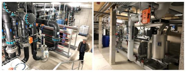
Figure 3. Left: 1 MW Heat pump; Right: Lake water pumping station. (Source: Corporation Weggis).
