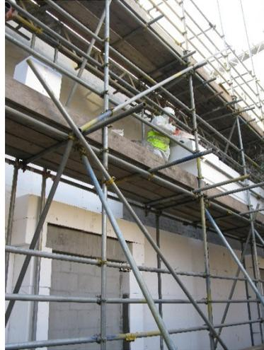
Figure I-7. 290 mm EPS above ground.
