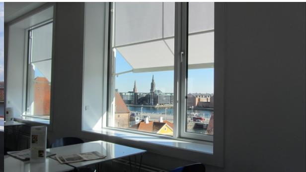
Figure B-28. Solar shading, adjustable vertical/horizontal.
