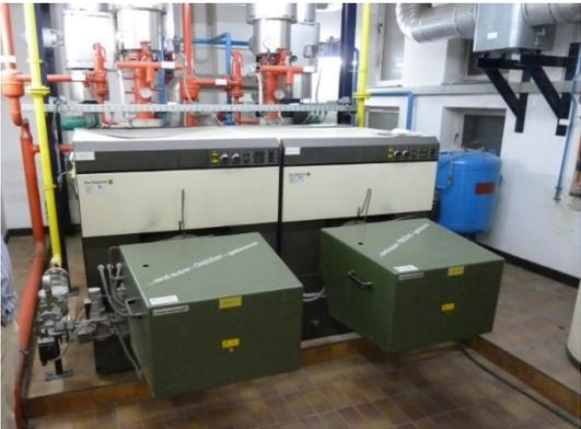
A photograph of the interior heating system, showing a large white boiler unit, green electrical control boxes, and various pipes and valves.                               |
