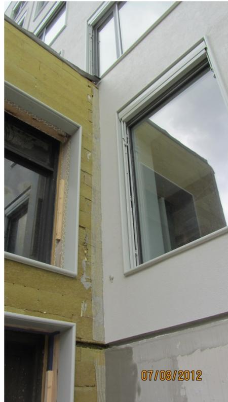
Figure B-26. Insulation and new windows installed.
