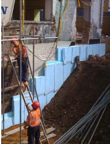
Figure I-6. 200 XPS below ground mineral wool.
