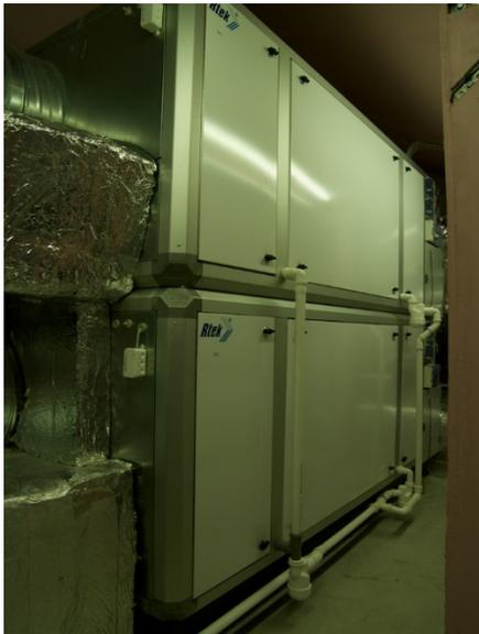
Figure C-12. Ventilation with heat recovery.
