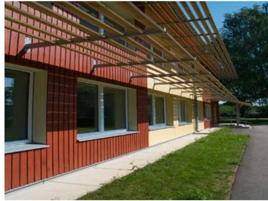
Figure C-6. After refurbishment – overhangs for summer heat protection.
