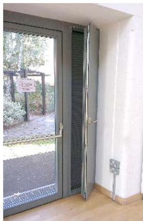
**Figure I-14. Manual air intake panel for secure night-purge ventilation.**
