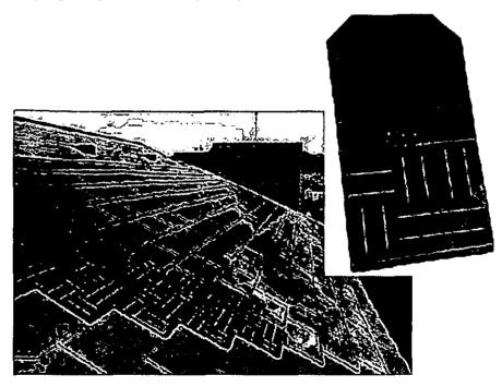
Figure 6.1 Photovoltaic cells installed as roof tiles
