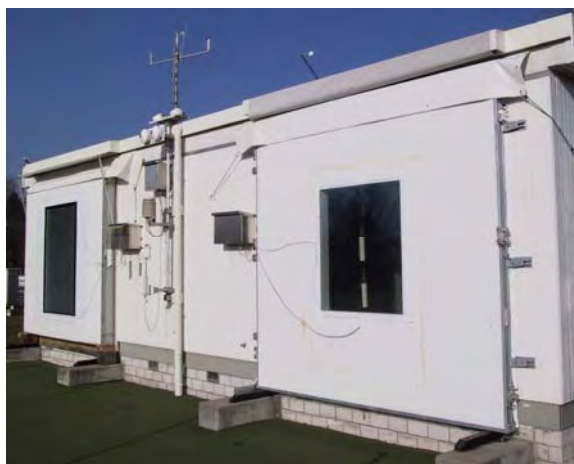
Figure 6.1. A photograph of the test cell.
