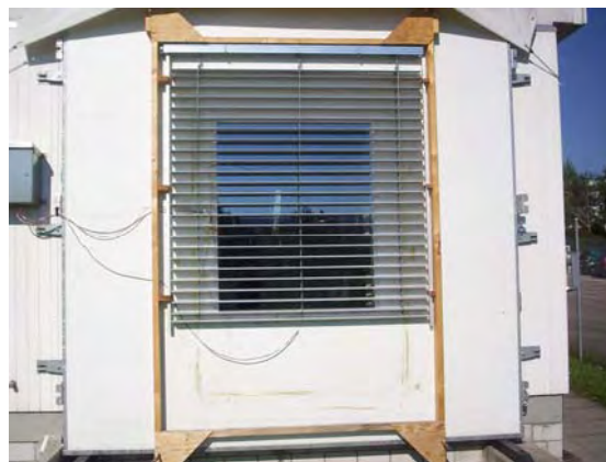
Figure 9.1. Photograph of the exterior blind mounted in front of the test cell.
