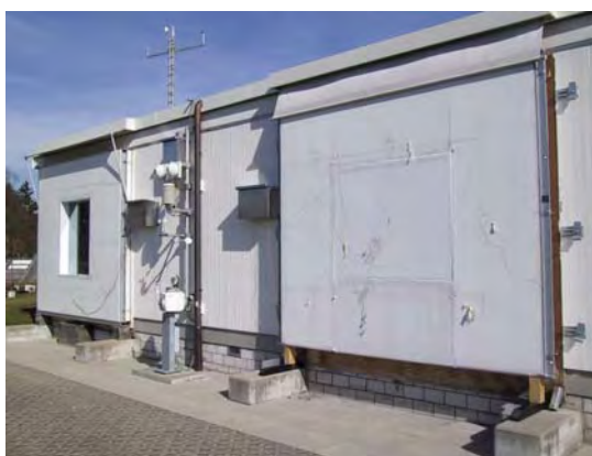
Figure 4.1b. Outdoor test facility with removable façade element.
