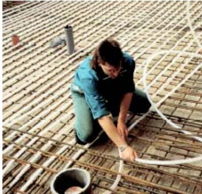
Installation of the pipes on the reinforcement grid of the future concrete floor slab (Hauser 2002)
