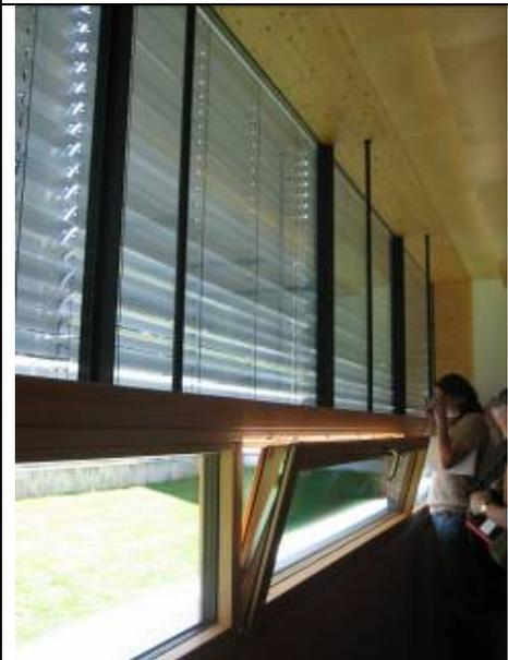
Picture of the façade in the classrooms. The external shading is automated, the automation can, however, be overruled by the users. Inlet openings are placed in the bottom in order to allow shading and ventilation simultaneously. The classrooms are also mechanically ventilated through inlet and outlet openings in the ceiling.
