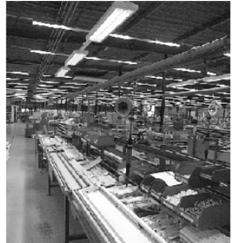
Increase in productivity and decrease in lighting energy consumption by task lighting and improved lighting control system
