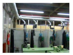
Figure 6.104. Demand-based local exhaust system for 24-work stations at the New England Institute of Technology.
