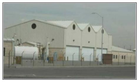
Figure 6.1. TEMF building at Fort Bliss with a reflective white metal roof.
