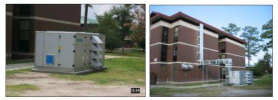
Figure 7.73. Blue rectangular opening is the location of (future) supply duct connection. Completed system is shown at the right.
