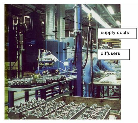
Figure 6.20. Industrial displacement ventilation system.
