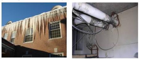
Figure 6.117. Cold climate exfiltration problems (left) and hot humid air infiltration problems (right).
