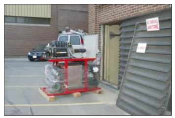
Figure 7.140. New chiller before installation at Newport RI.
