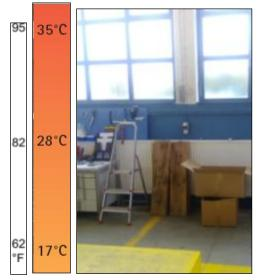
Figure 7.126. Radiators were used for heating prior to the retrofit; as a result, temperature varied greatly between the floor and ceiling.
