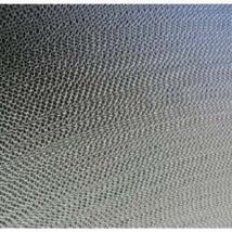
Source: <u>www.xetexinc.com</u> Figure 6.33. Densely packed fins of a rotary heat exchanger.
