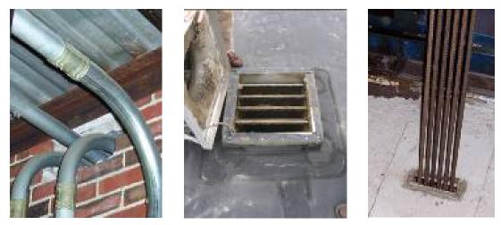
Figure 6.119. Unsealed penetrations (left); open louvers to vent shafts (middle); elevator cable holes can be made tighter (right).
