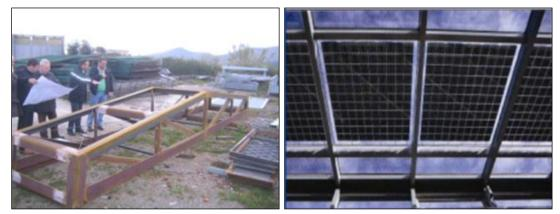
Figure 7.116. Structure for the glazed roof and semi-transparent PV cells.
