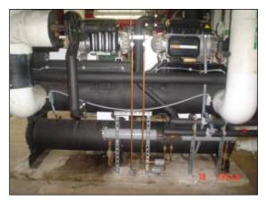
Figure 7.139. Oil-free magnetic bearing chiller compressor.
