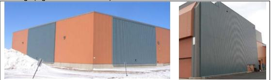
Figure 7.134. SolarWall panel colors were selected to enhance building appearance.
