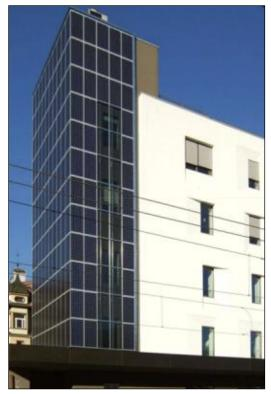
Figure 7.14. View of the PV cells installed on the tower.
