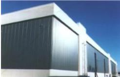
a. Typical Industrial Application Figure 6.79. Transpired solar wall applications.
