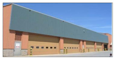
Figure 7.129. Unglazed SolarWall panels installed above rollup doors of a maintenance shop, Fort Drum, NY.
