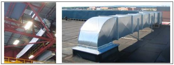
Figure 7.133. Ventilation air distribution ducting.
