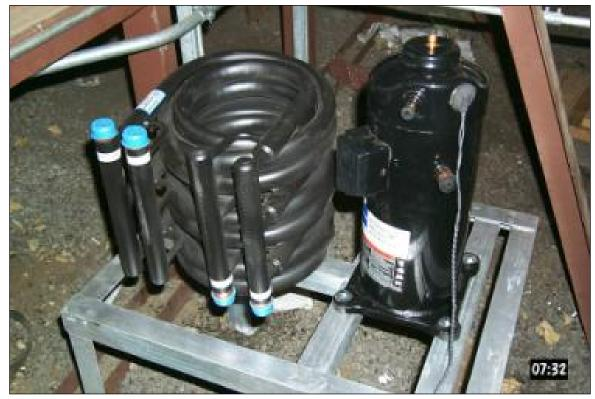
Figure 7.55. DX compressor and water-cooled condenser.
