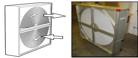
Source: <u>www.xetexinc.com</u> Figure 6.32. Rotary heat exchanger.
