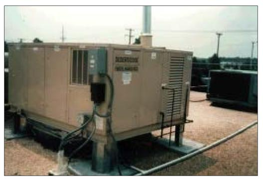
Figure 7.39. Engelhard/ICC two-wheel desiccant systems (TWDS) rooftop unit.
