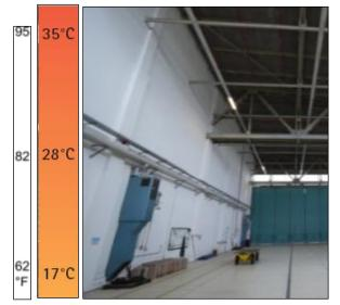
Figure 7.104. A forced-air system was used to heat the hangar.
