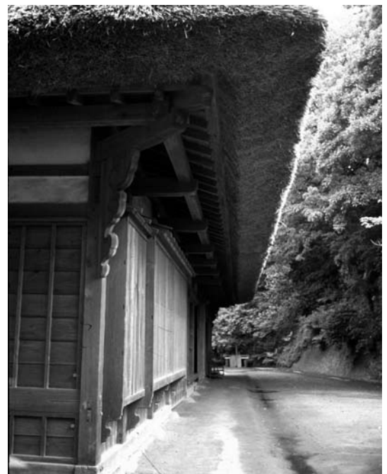
Fig. 6: A Japanese vernacular house with thatched roof. A bunch of dried straw having hollow space filled with air plays a key role on controlling the indoor environmental condition.
