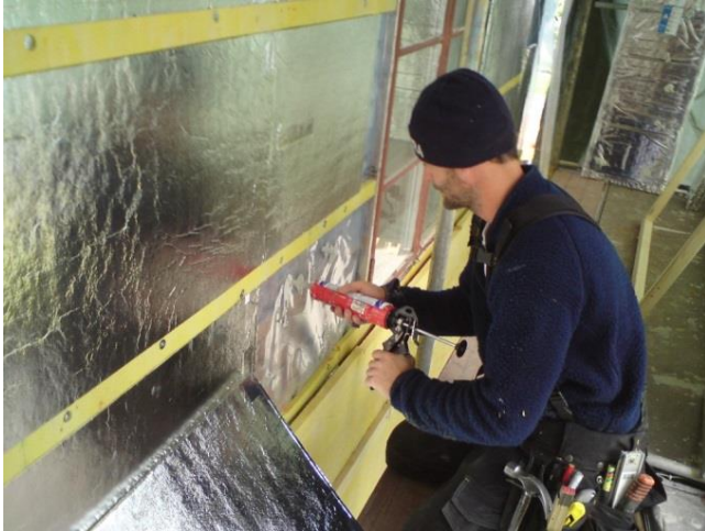
Figure 6.6: Retrofitted wall with 20 mm VIP covered by 30 mm glass wool boards. Between the VIP are 20x50 mm strips of high density glass wool attached to allow attachment of the wooden cover boarding. Photo: Pär Johansson.
