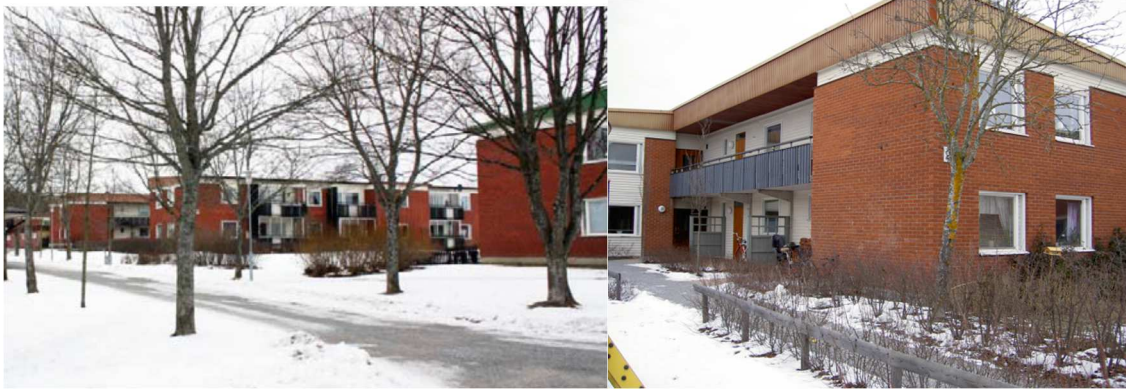
Figure 2.25 Overview of the area with the studied building.
