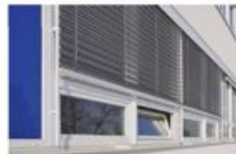
Figure 6: Exterior sunblinds installed on the windows of all classrooms. [2]
