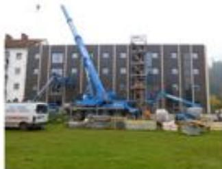
Figure 7: assembling of the prefabricated façade elements
