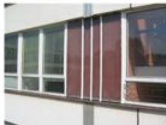
Figure 13: Original state: Row of windows separated by particle-board panels where interior walls connect to the façade. [2]
