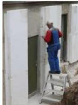
Figure 4: Insulation work on the basement walls
