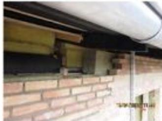
Figure 7: New insulation and new bricks near the roof
