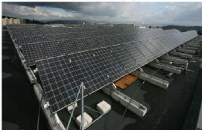
Figure 11: Photovoltaic power plant on the roof of the school's main block. [3]
