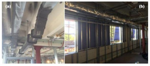
Figure D-9. Ductwork joint seals (a) alone that did not meet DALT criteria; insulation provided (b).
