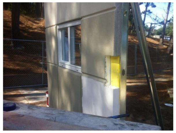
Figure D-7. PDQA process deliverables such as window mock-ups can be effective QA tools when used correctly.
