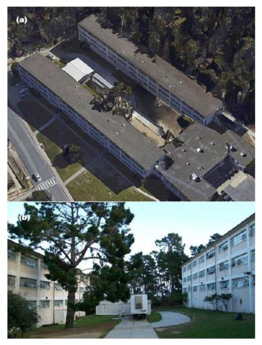
Figure D-1. (a) Bldg. 630's 3-story barracks wings (1-story connecting structure is administrative spaces that are not part of the case study), (b) uninsulated concrete masonry unit (CMU) walls and single-pane windows—typically left open year-round for ventilation—make for poor building envelope performance.
