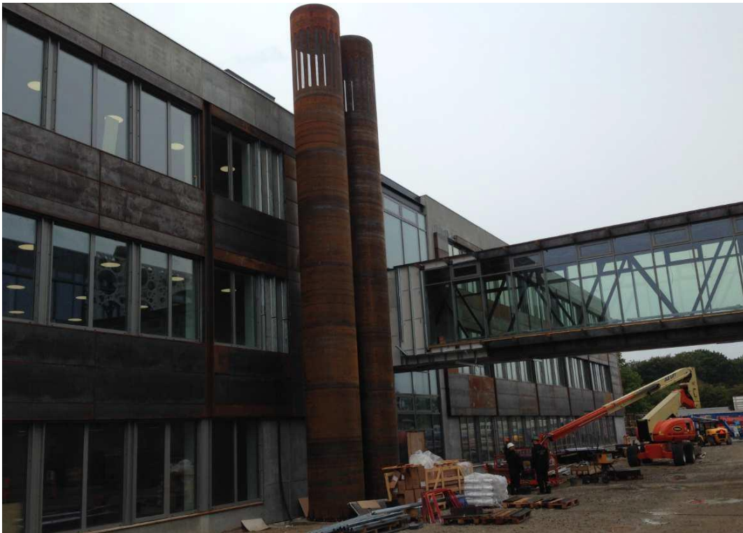
Figure 4.3 Air intake chimneys for ventilation systems (construction phase).
