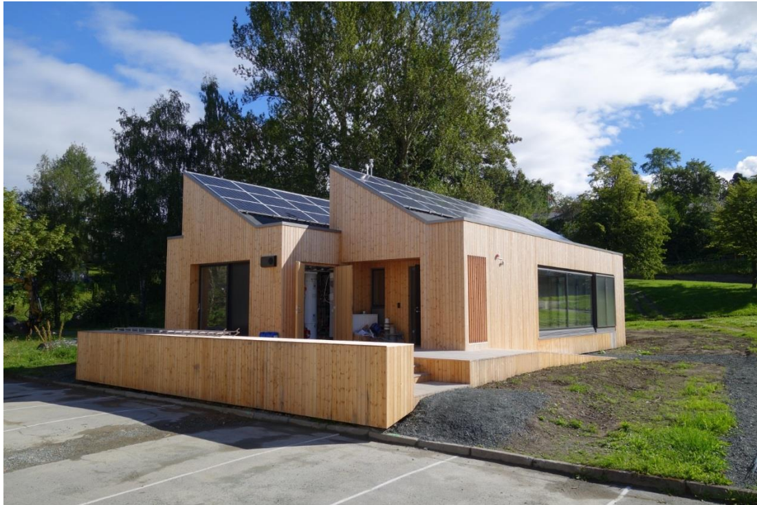
Figure 5.3. The Living Lab house at NTNU/SINTEF, Norway (Annex 67, 2016).
