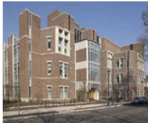
Office building A, USA 6425m 2 , 364kWh/m 2 ·a
