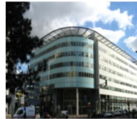
Office building, Lyon 17k m 2 , 165kWh/m 2 ·a
