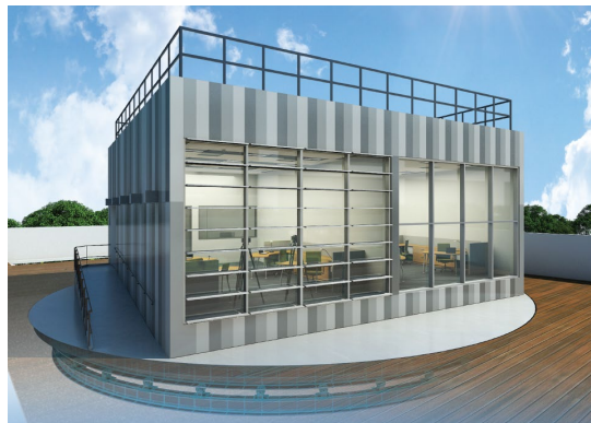
Figure 9-1 BCA’s Skylab in Singapore (a rotatable test facility) https://www1.bca.gov.sg/buildsg/sustainability/bca-skylab
