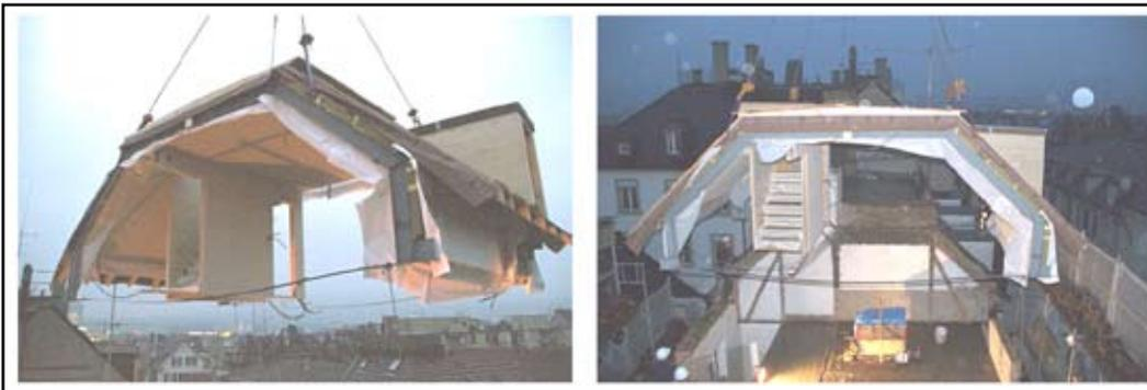
*New roof elements are lifted onto the building. The new roof is completed within hours.*
