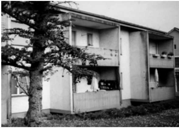
Figure 8: Retrofit Demonstration Building Therwil in Switzerland, After renovation (right) only 1/4 of the original energy consumption (left) for heating and hot water (~ 50 kWh/(m 2 -a) is consumed.
