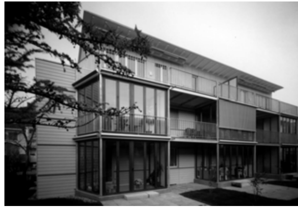
Figure 8: Retrofit Demonstration Building Therwil in Switzerland, After renovation (right) only 1/4 of the original energy consumption (left) for heating and hot water (~ 50 kWh/(m 2 -a) is consumed.
