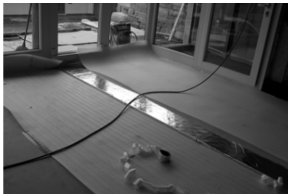
Figure 10: Vacuum insulation is a new technology and due to its very low space demand especially suited for building renovation.
