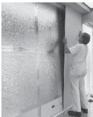
Figure 10: Vacuum insulation is a new technology and due to its very low space demand especially suited for building renovation.
