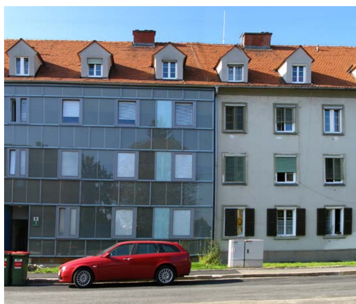
Figure 3. Refurbished row house at Dieselweg in Graz (left) and original situation (right).
