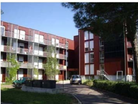
Figure 1: South view of the building after retrofitting
