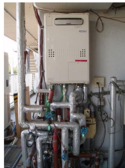
Figure 2. Condensing boiler under test.
