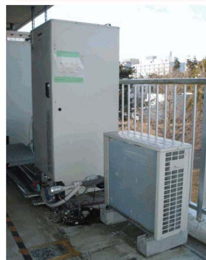
Figure 3. EcoCute - heat pump domestic hot water system.
